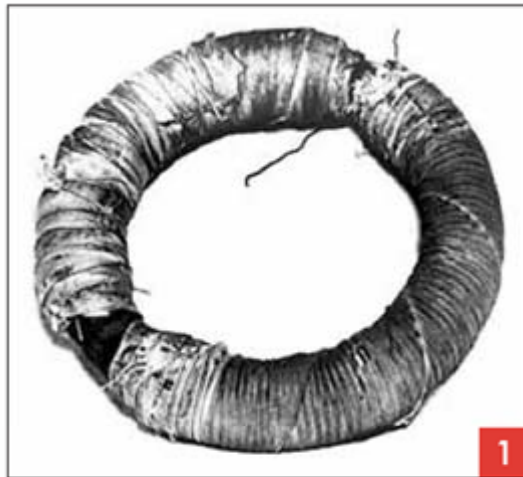
Photo of Faraday's original transformer (courtesy MIT Burndy Library).
